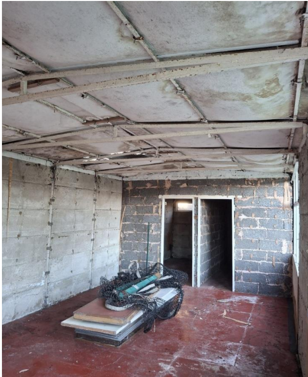
Picture 5: Stripped out interior
