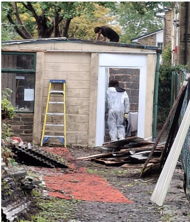
Picture 7: Roof material ready for removal
