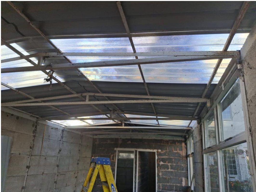
Picture 8-9: The new metal roof from inside and outside with skylights for improved light
