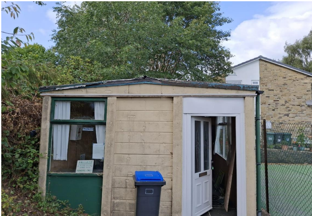
Picture 1-3: The St Peter's Clubhouse before the new roof, outside and inside
